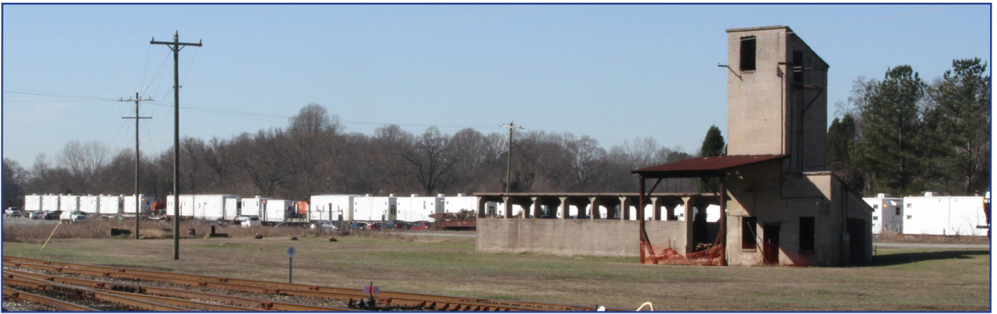
Part of the NS work train consist residing on the NCTM grounds: three of the cars are converted box cars.
