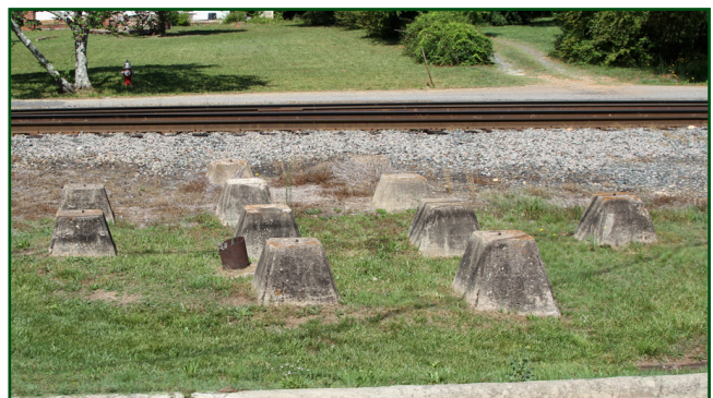
FOOT PRINT FROM THE PAST: the foundation piers of the old Norfolk Southern water tank from the steam era is still present in Star.
